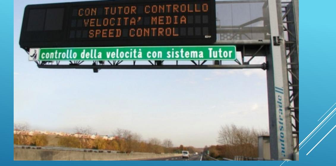
The Speed Control with Tutor System can measure the "instant" speed as the vehicle passes or they can average the speed of the vehicle in a stretch of road between two detection stations.
